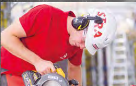
// Concrete Construction / Betonbau
